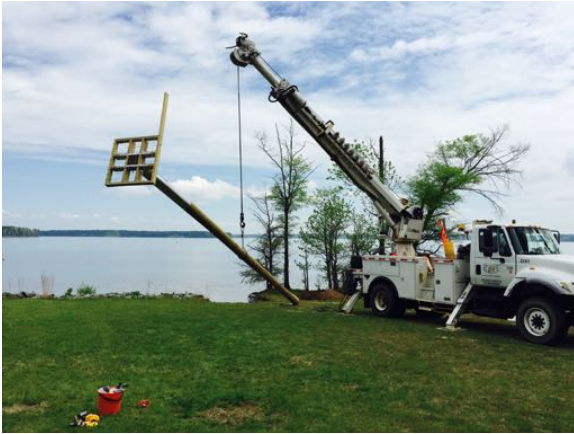
Osprey Nest being installed by Duke Energy
