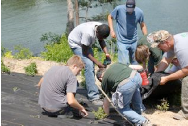
Putting the Erosion Barrier Down
