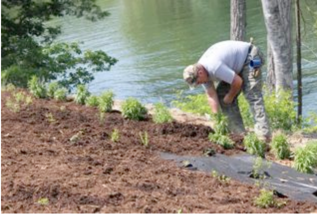
Spreading the Mulch
